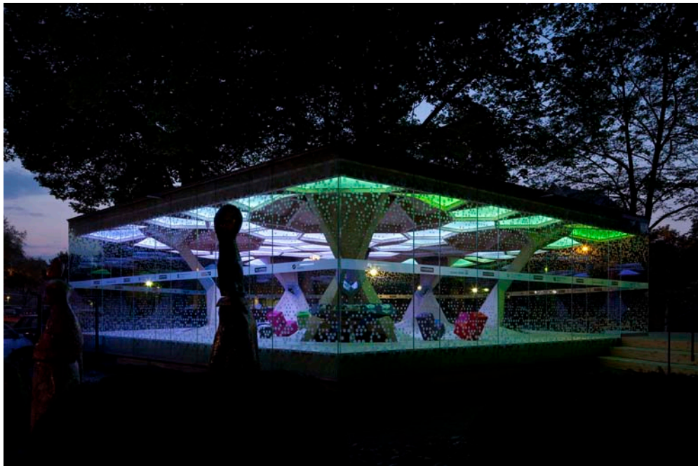
Figure 3. The pavilion and the interactive light installation at night (Photo by Roland Borgmann).
